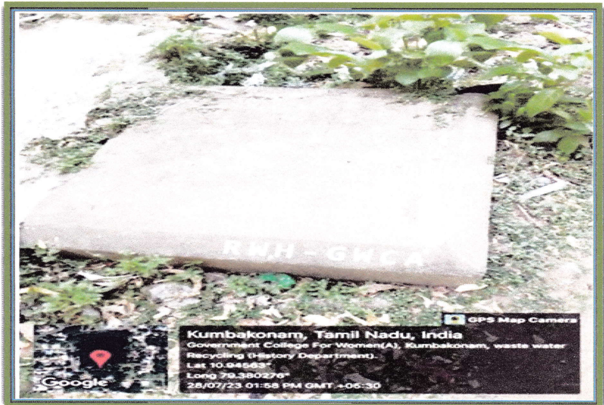
Rain water Harvesting
